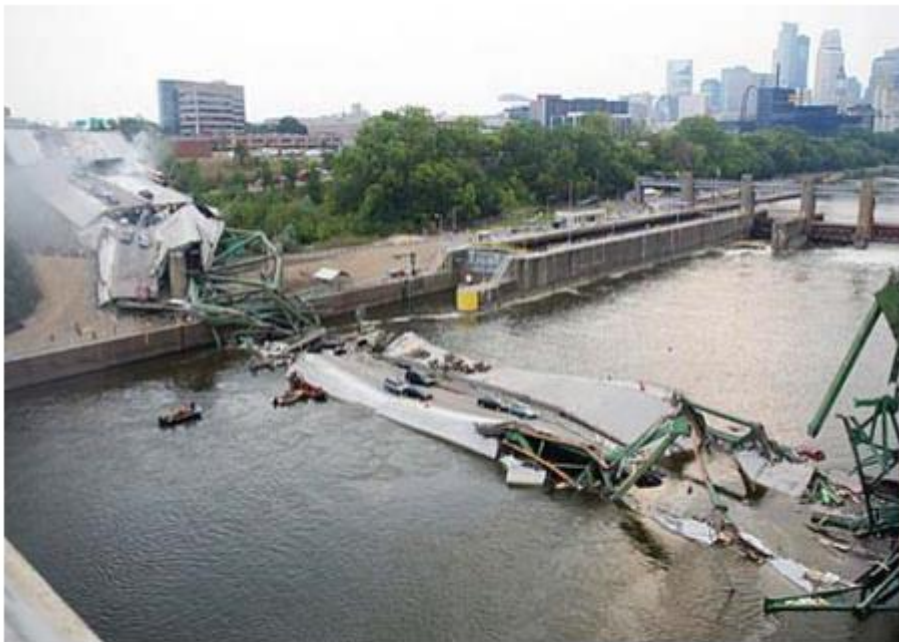
Fig. 2 Collapse of Bridge on Mississippi River
